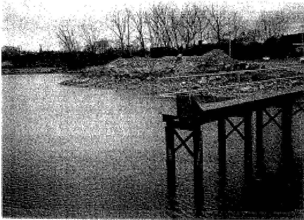
4.) LOOKING SOUTHEAST FROM THE BULKHEAD AT THE SHORELINE WHERE NEW TRAVELLIFT PIERS WILL BE BUILT. 03-09
