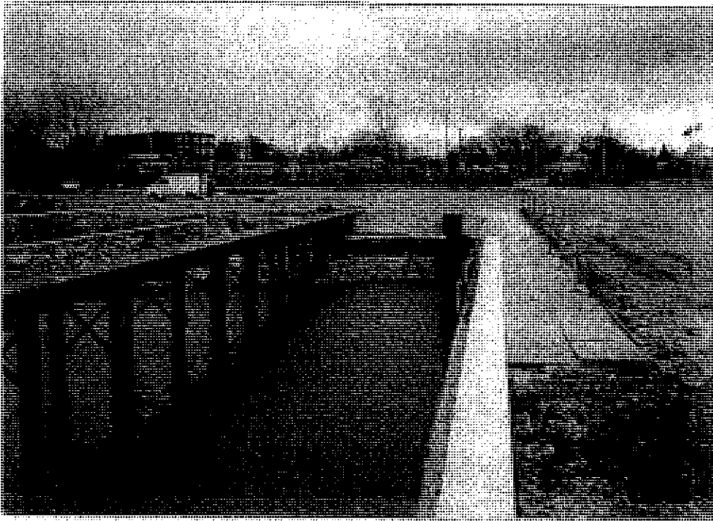
3.) LOOKING SOUTH ALONG THE BULKHEAD AT THE EXISTING TRAVELLIFT PIERS. 03-09
